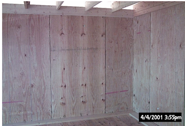
Overall View of Retrofitted SEA Hut
