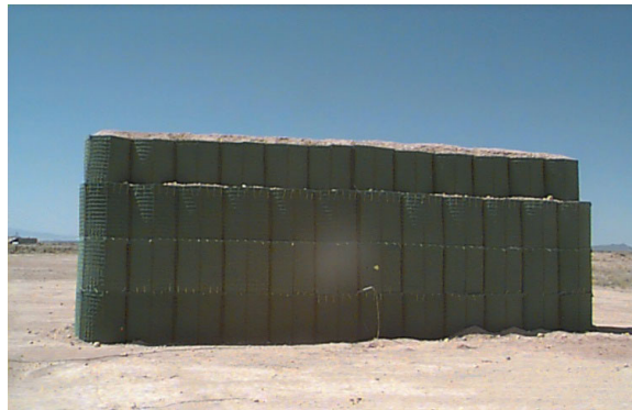
Figure 22: Earth Filled Barrier
