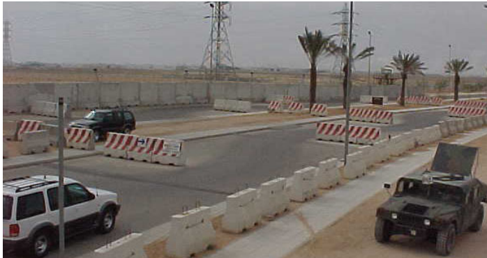
Figure 24: Jersey Barriers Employed for Countermobility
