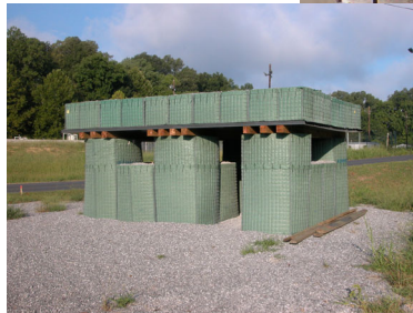
Figure 28: Concertainer Styled Barriers Used as Blast Walls and Fighting Positions (Concertainer Construction Techniques per ERDC Guidance)
