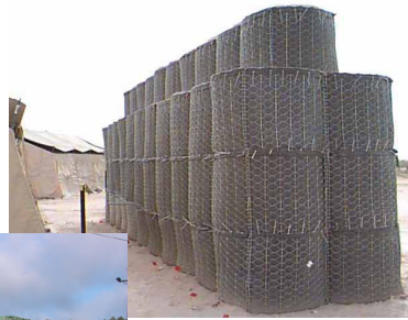
Figure 28: Concertainer Styled Barriers Used as Blast Walls and Fighting Positions (Concertainer Construction Techniques per ERDC Guidance)
