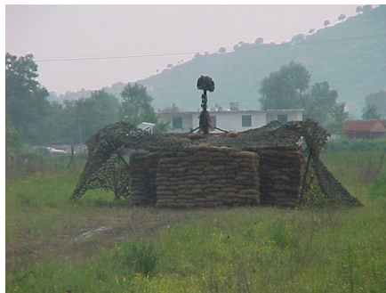
Figure 26: Sandbags Used for Fragment Protection
