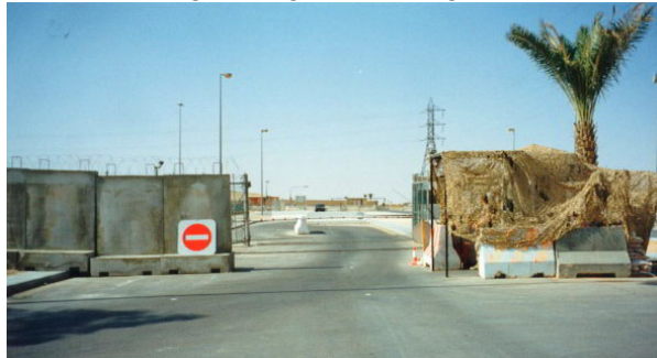
Figure 25: Bitburg Barriers Employed for Countermobility
