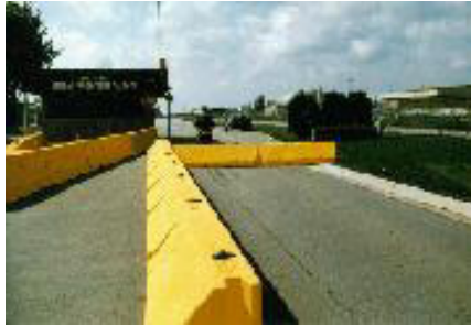
Figure 27: Water Filled Barriers Used for Countermobility
