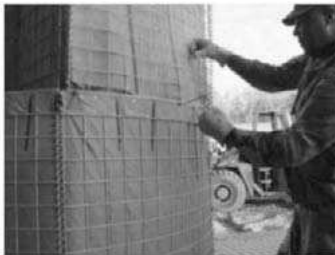
Connecting second layer to first using plastic wire ties
