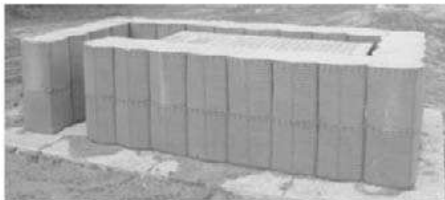
Second layer in place and filled
