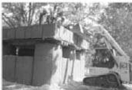
Placing soil cover on top of bunker
