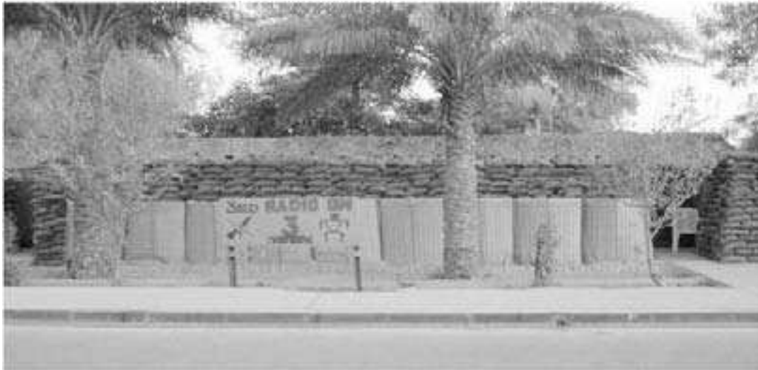
Figure 8-1. Example of providing full-height sidewall protection
