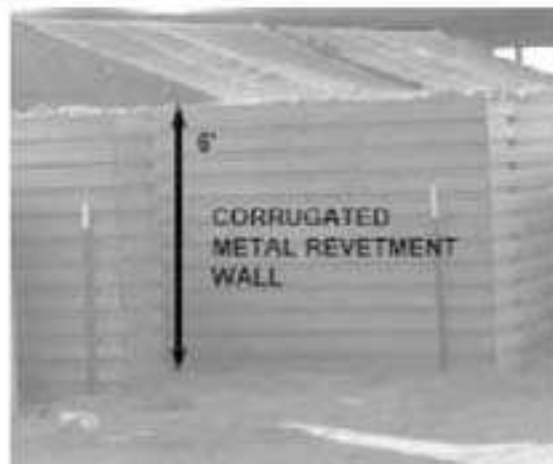
Figure 8-9. Metal bin revetment used for sidewall protection
