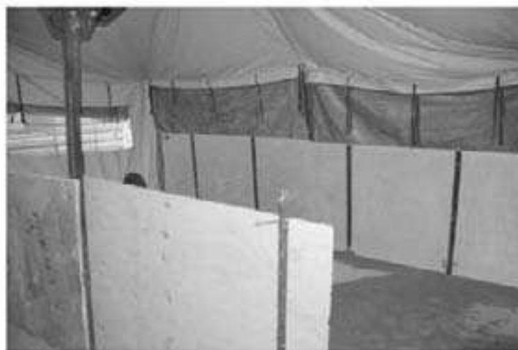
Figure 8-16. Use of E-glass and U-pickets for low-height protection.
