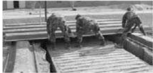
Place sheet piling roof
