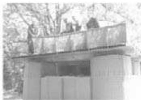
Placing Concrete container around roof perimeter
