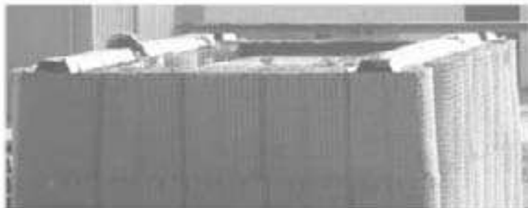
Sheet piling in place on side walls
