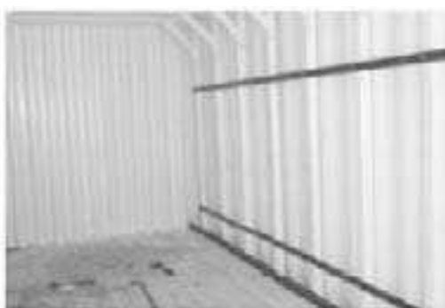
Flat bar straps attached to frames
