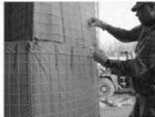
Connecting second layer to first using plastic wire ties
