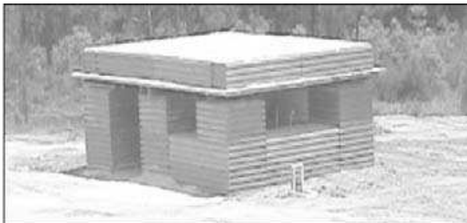
Figure 8-75. Aboveground Metal Bin Large Observation Post
