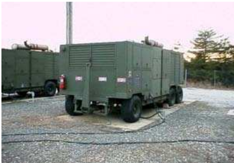
Figure 11-2. Prime Power generator
