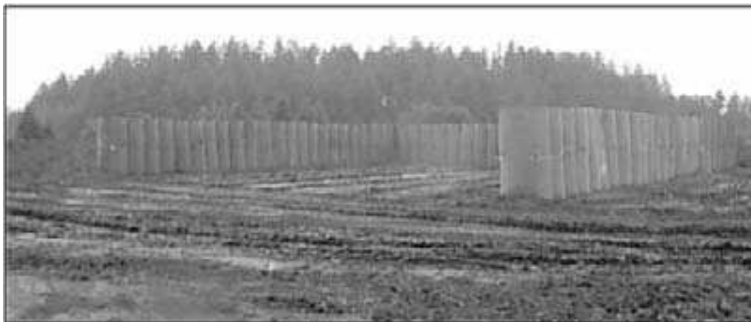
Figure 8-17. Hesco revetment design for helicopter protection
