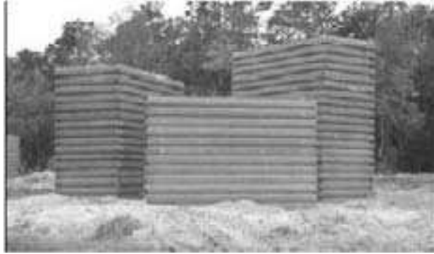
Figure 8-8. Examples of corrugated metal bin revetments
