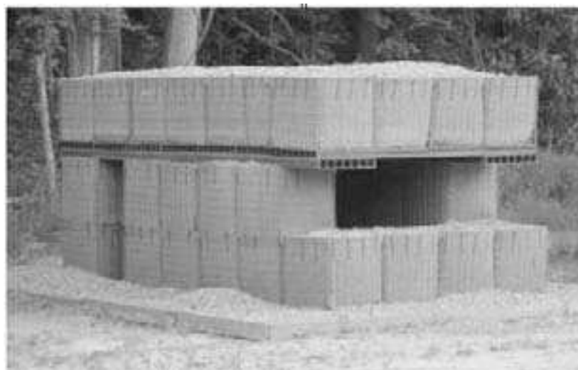
Figure 8-88. Improvised above-ground, single-bay fighting position with Composolite® roof
