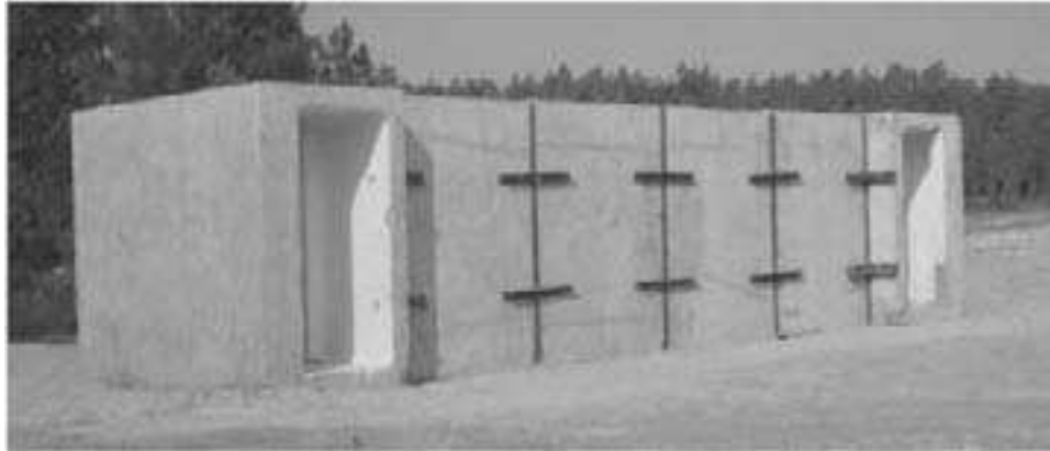
Figure 8-37. Basic Modular Concrete Bunker (without soil cover)
