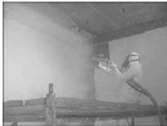
Figure 8-93. Spray-on polymer retrofit system
