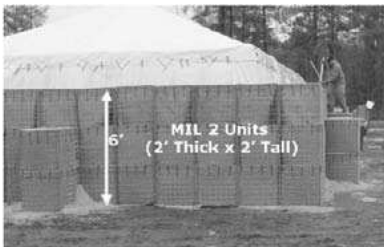
Figure 8-5. Mil 2 Hesco Bastion soil-filled wall
