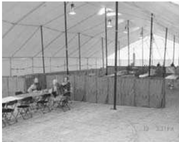
Figure 8-26. Example of Hescos used to compartmentalize
