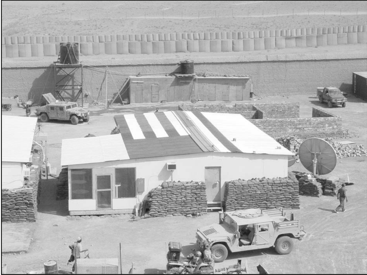
Figure 2-10. Sandbags stacked chest-high around tactical facility structures
