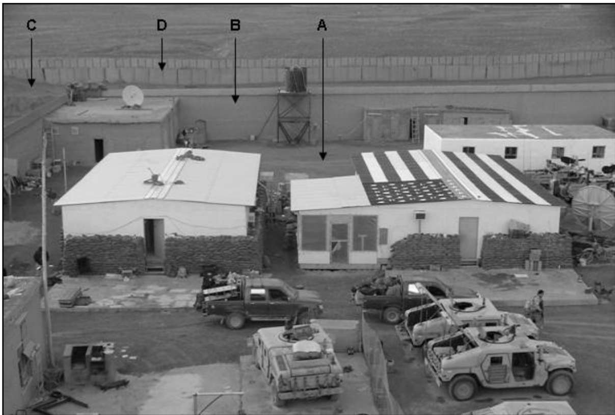
Figure 2-2. Rural Special Forces tactical facility overview (example 2)
