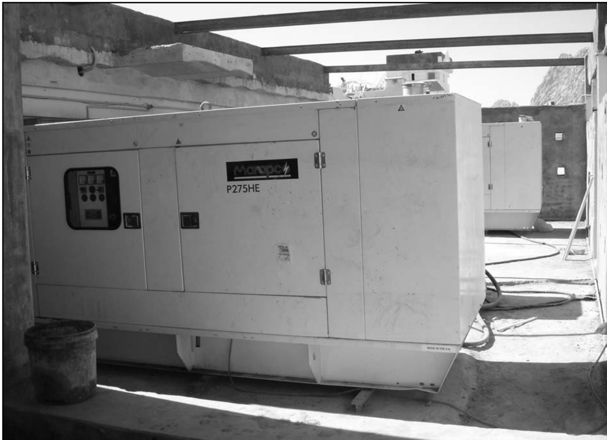
Figure 1-10. Redundant permanent phase generators
