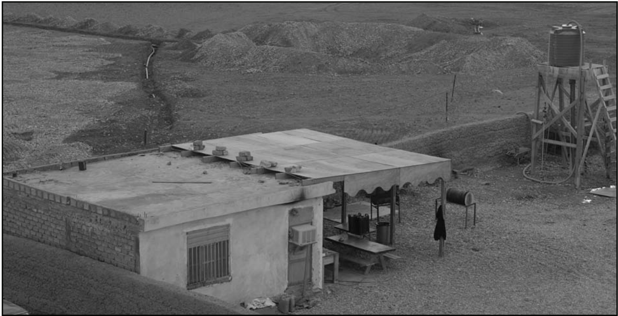
Figure 2-3. Inner protective berm
