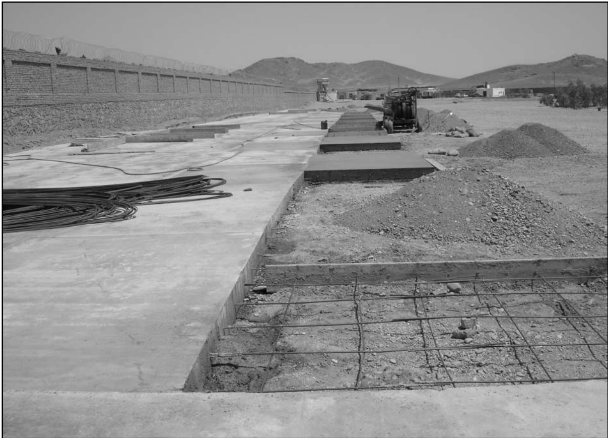
Figure 2-15. Constructing a rebar reinforced concrete helicopter pad
