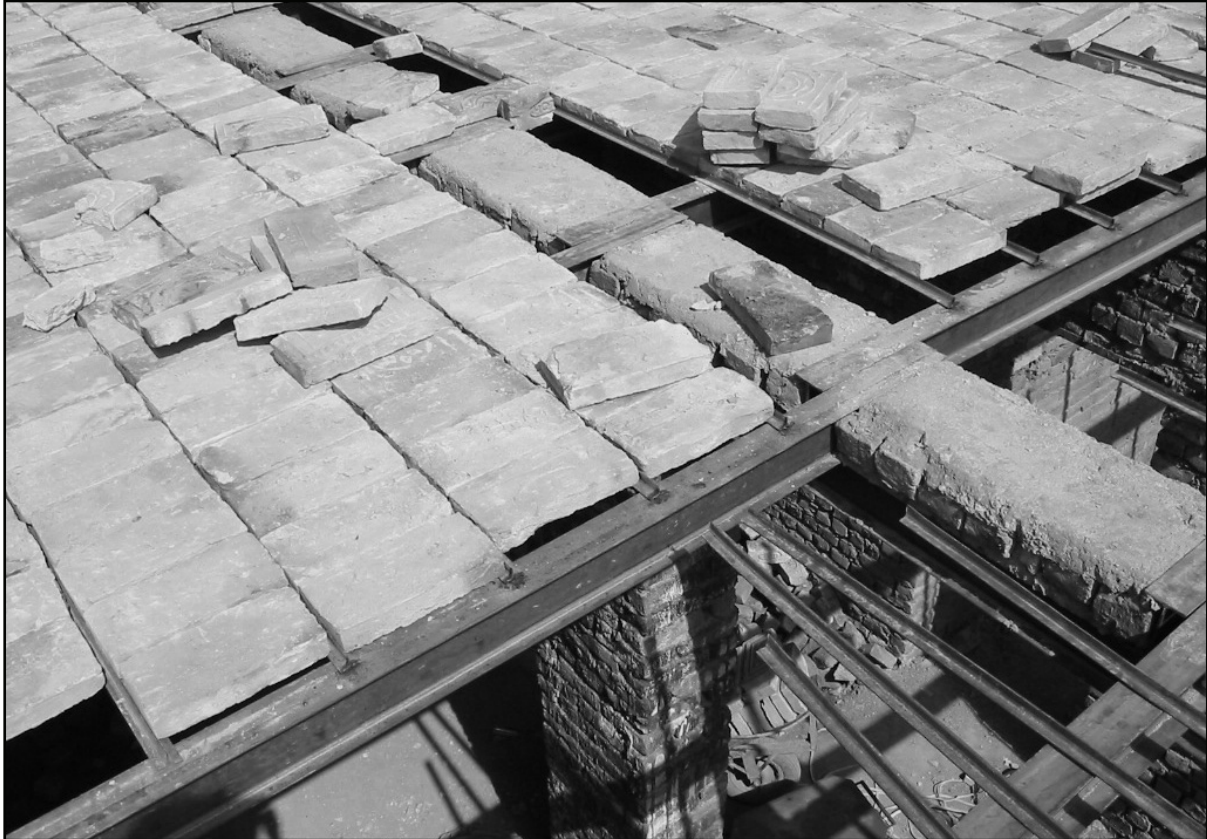
Figure 3-5. Brick slab roofing
