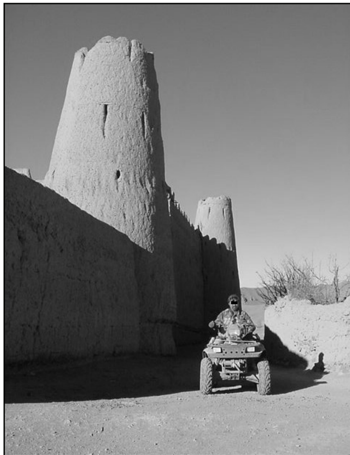
Figure 1-12. Tactical facility improved protection measure—solid, defensible mud wall
