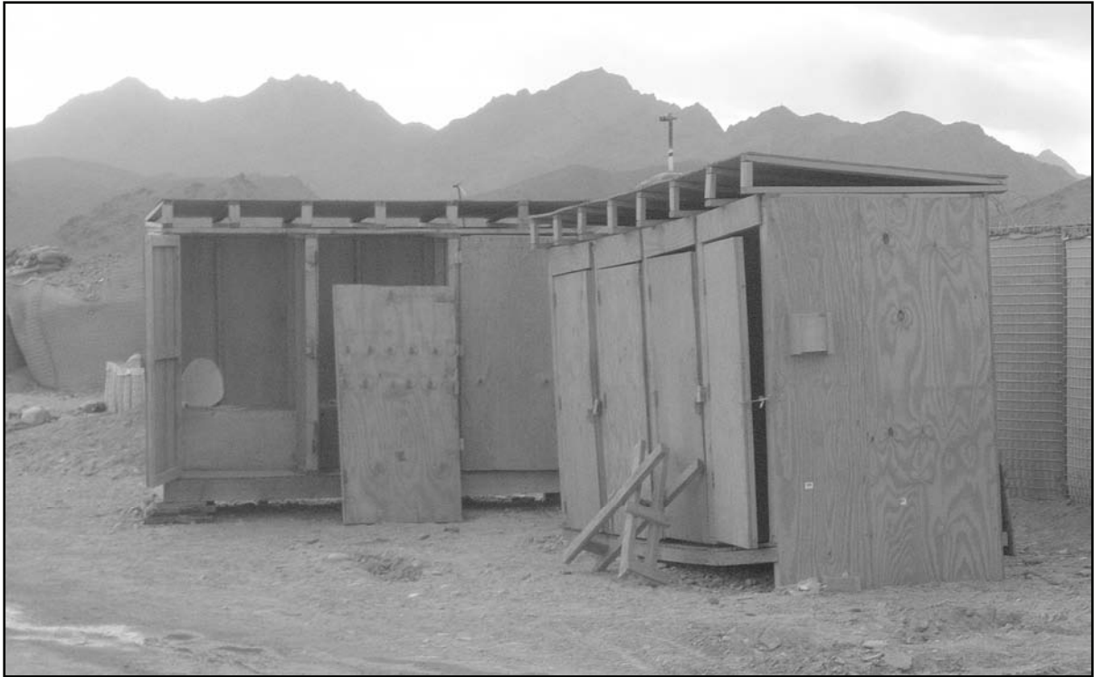
Figure 1-8. Temporary phase latrines
