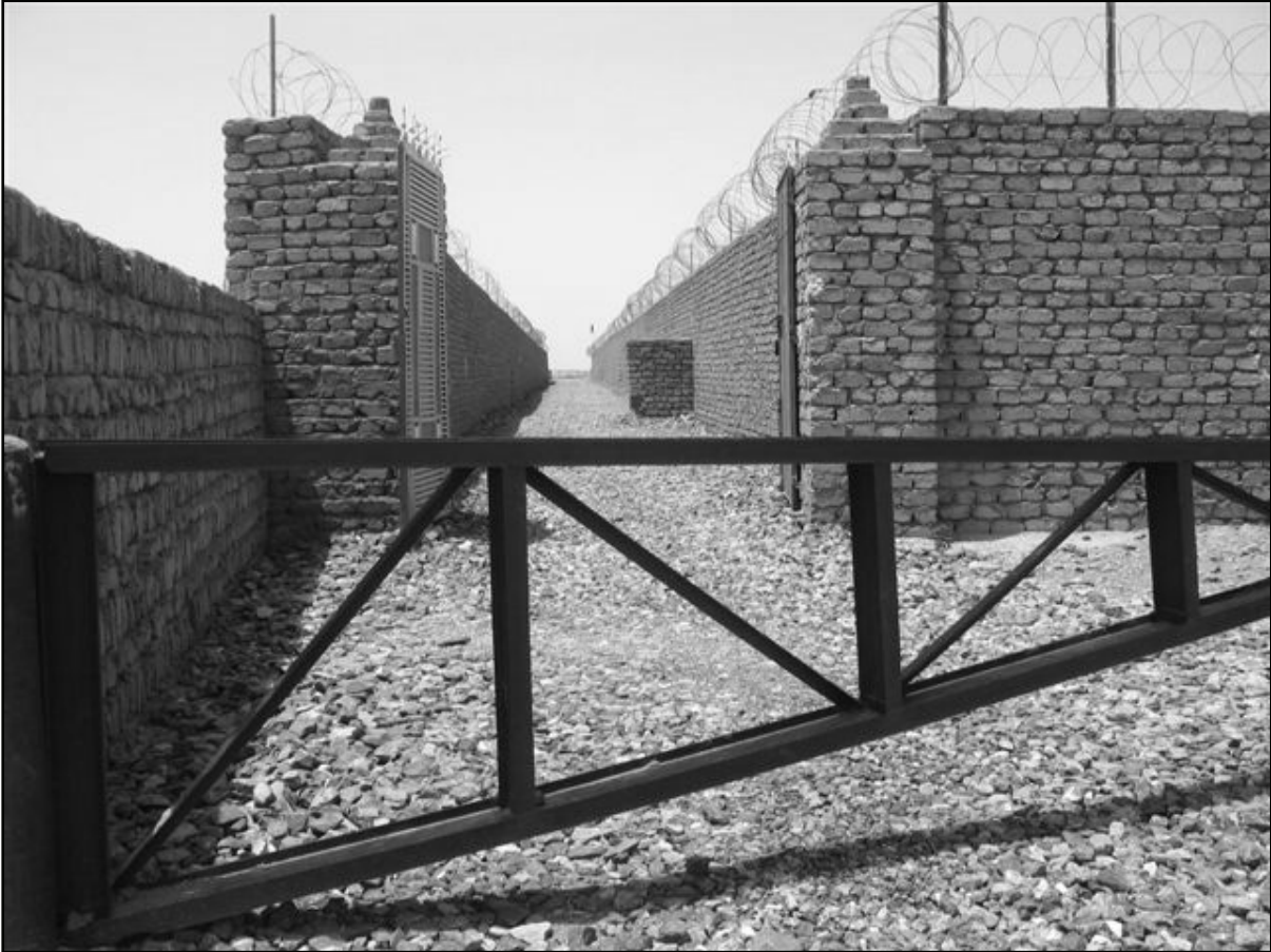
Figure 2-17. Main gate entrance and confinement zone
