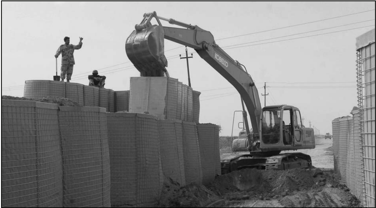
Figure 1-11. Filling stackable barrier systems
