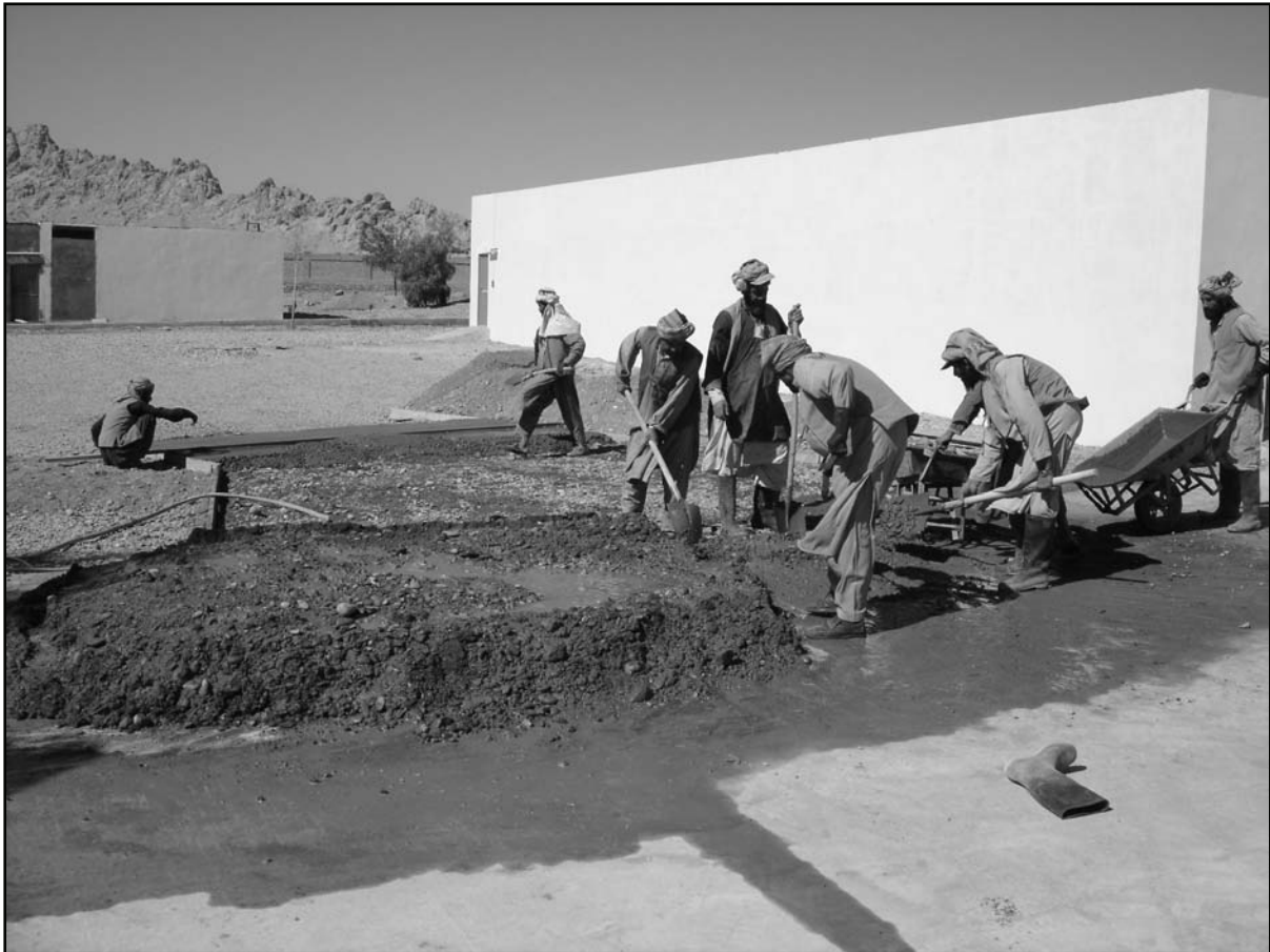
Figure 3-4. Indigenous employees mixing cement
