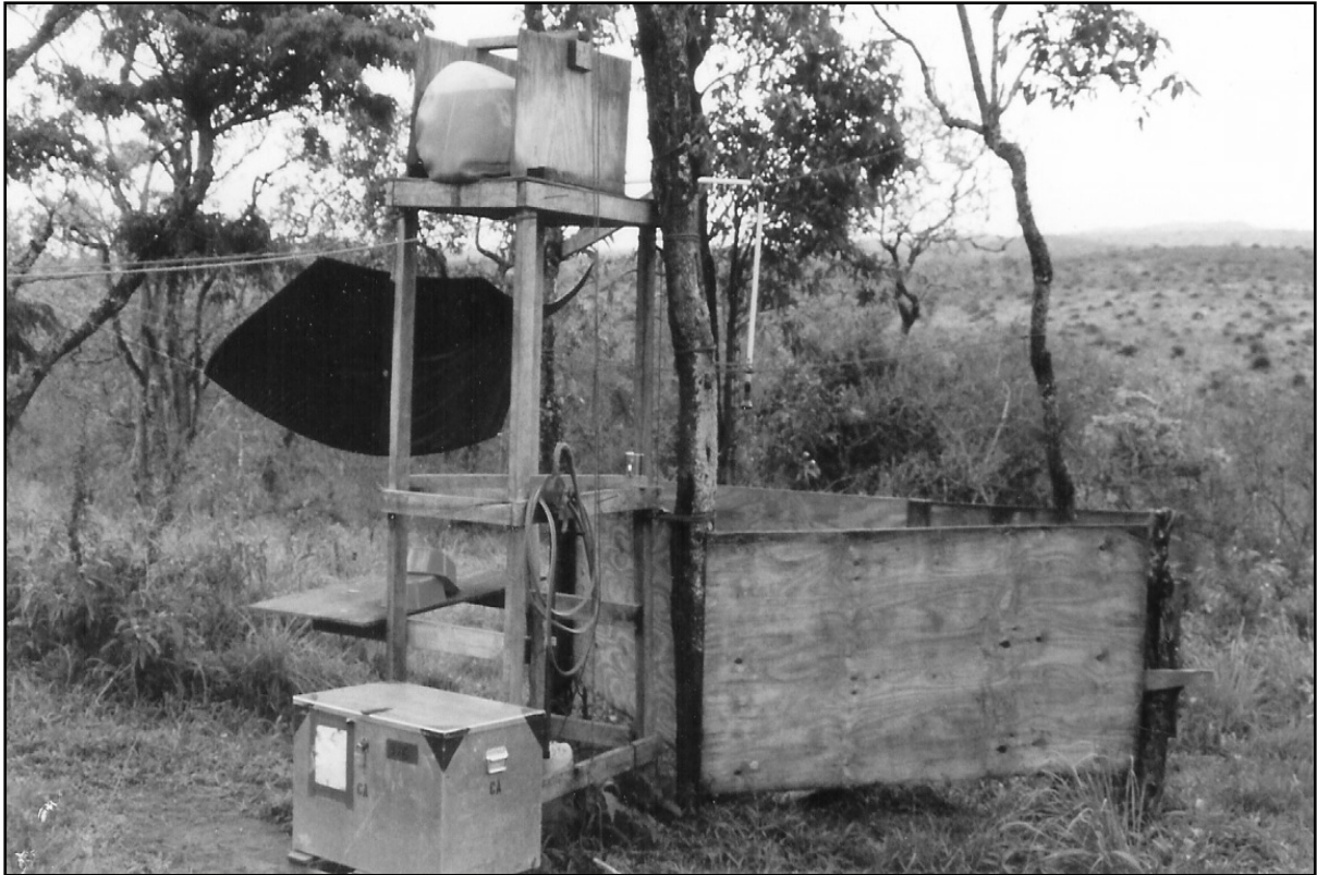
Figure 1-5. Initial phase rural tactical facility shower facility
