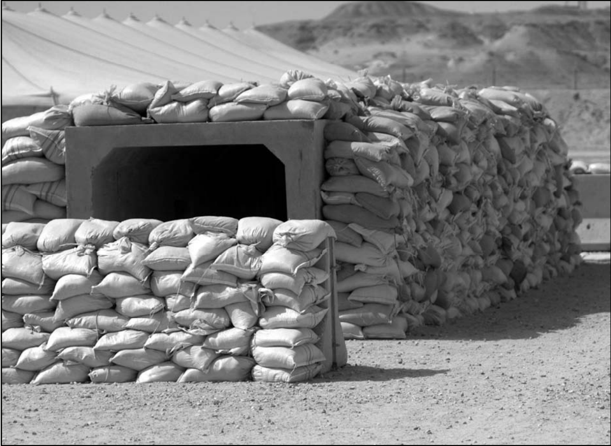
Figure 2-7. Personnel bunker offering indirect-fire protection
