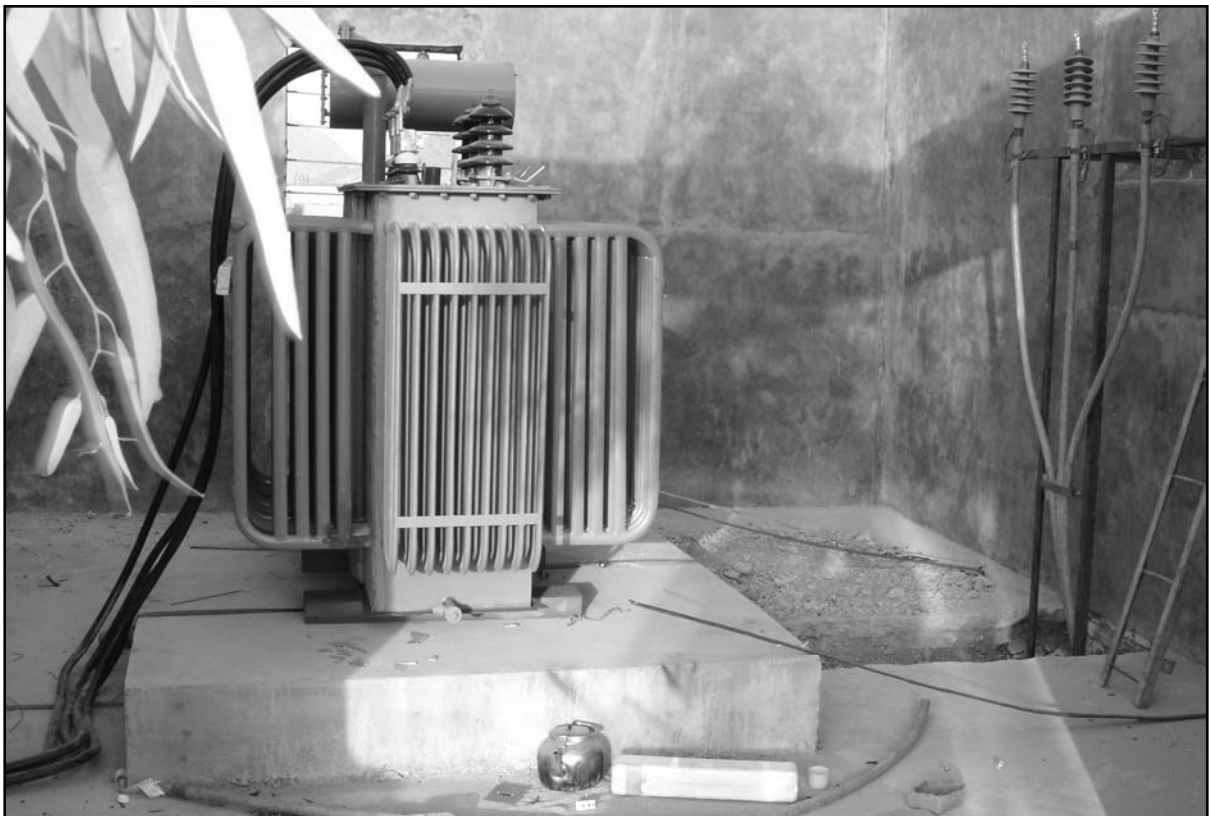
Figure 1-9. Power transformers routing electricity to structures
