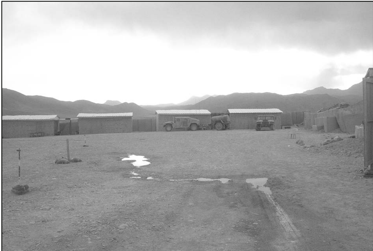
Figure 1-7. Temporary phase rural tactical facility wood-framed structures
