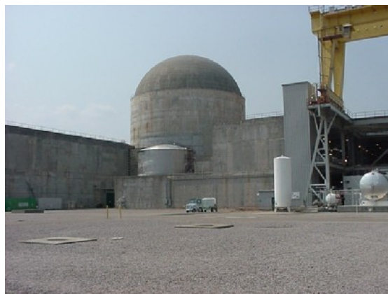
Figure 4 Nuclear Reactor Containment Building
